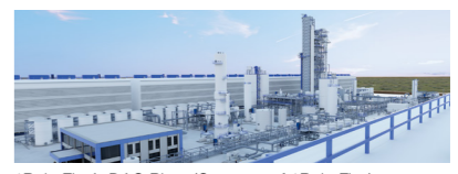
1PointFive's DAC Plant (Courtesy of 1PointFive)
